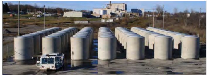
Top photo: 56 loaded NAC WVDP cask systems on West Valley storage pad. Right Photo: NAC WVDP storage cask being moved to storage pad
